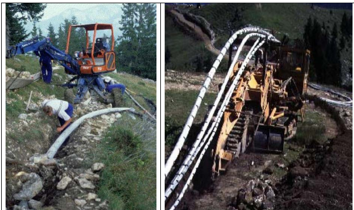
Figure 6.22: Installation of a pipe to discharge wastewater down to the valley to a municipal wastewater treatment plant, (BLU, 2000)
