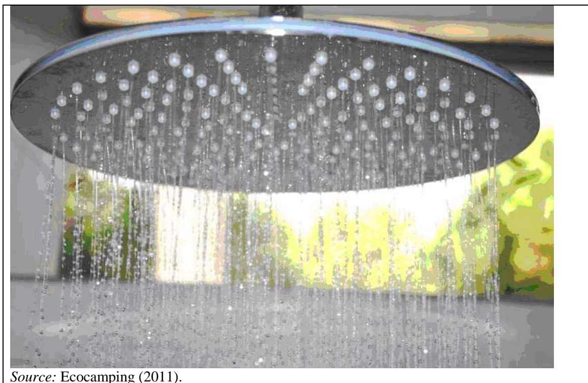
Figure 9.24: Example of a luxury low-flow rain-type showerhead installed in a luxury campsite, with a flow rate of 7 – 8 litres per minute
