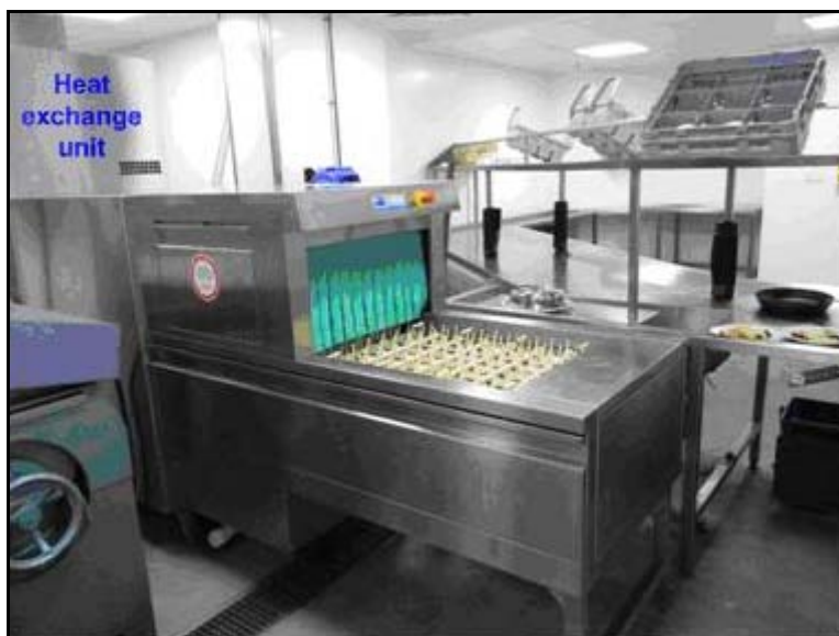
Figure 8.20: A conveyor-type dishwasher with heat recovery installed in The Savoy
